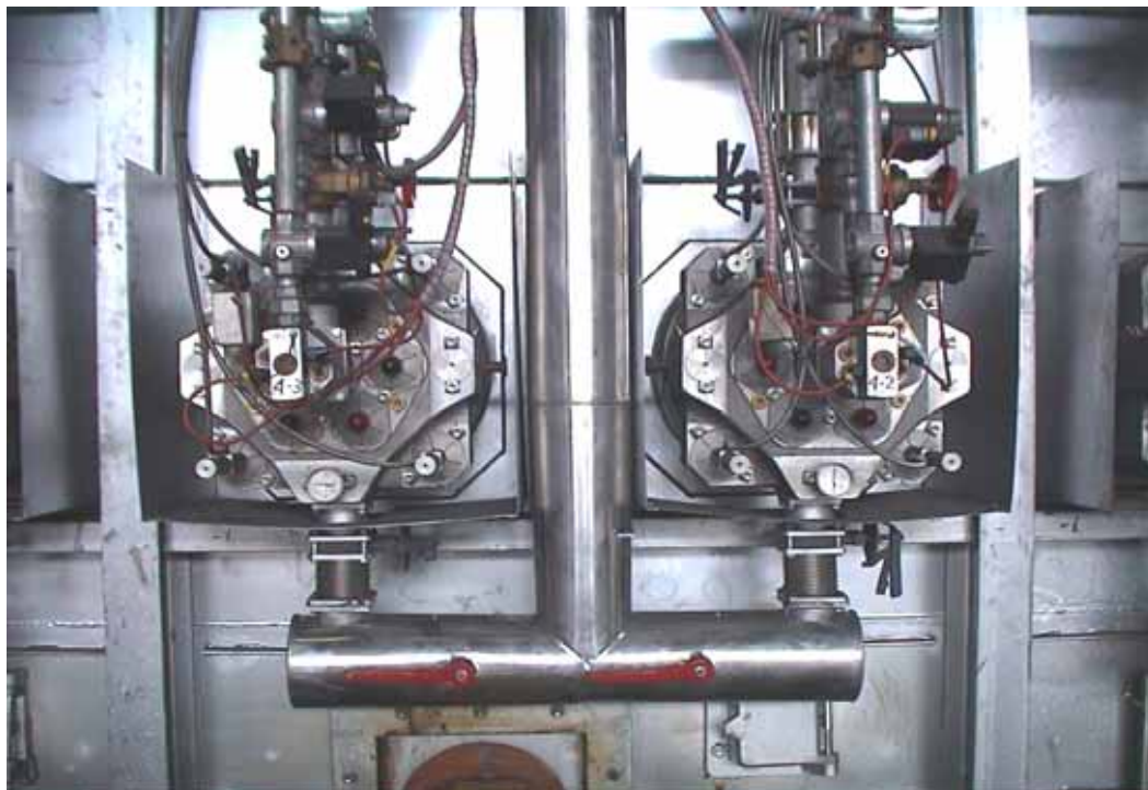
Figure 5 – Two Regemat® burners in operation
