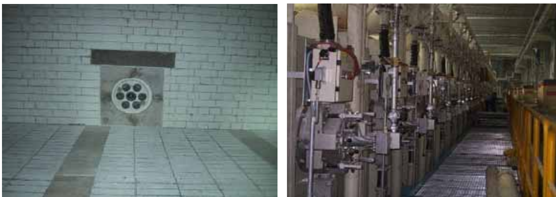
Figure 6 – Inside and outside view of the A&P Line (courtesy of KTN [3])
