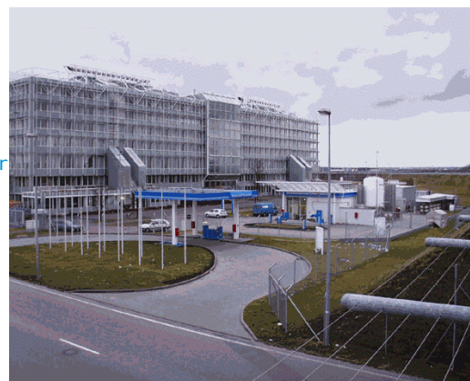
Figure 18: FLOX ® Reformer at the Munich Airport hydrogen fuel station
