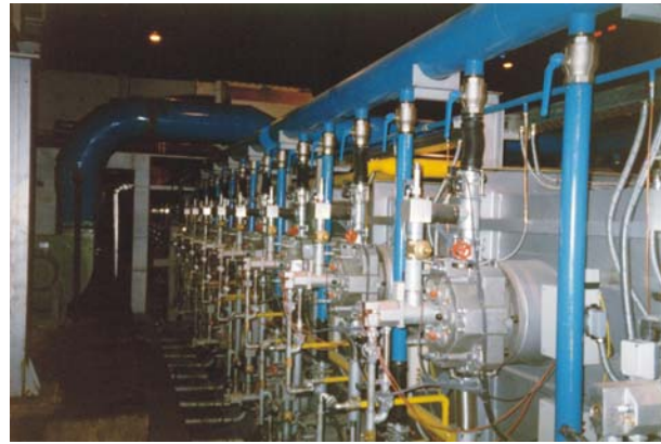
Figure 14: annealing and pickling line in Terni
